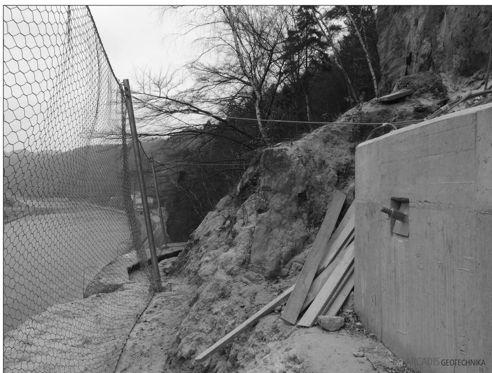
Fig. 3. Concrete frame, wall clamp and dynamic barrier in Hřensko (Photo: Arcadis GT a.s., 2012).
