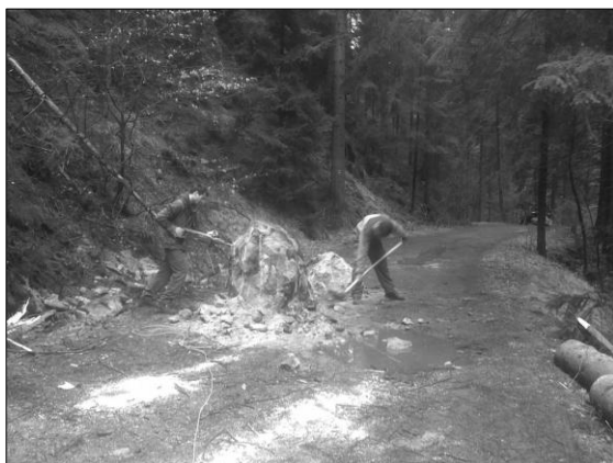
Fig. 1. Small rockfall at Kyjov, 1 \text{ m}^3 (Photo: J. Šafránek, 2012).
